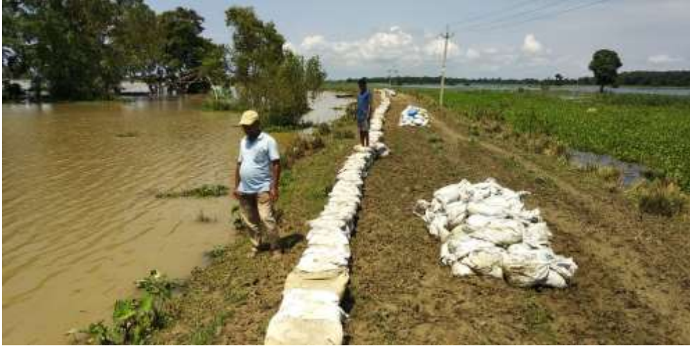
Figure 6: (c) current situation of E-10 (Dehing bund from Bhogamur to Sessamukh)
