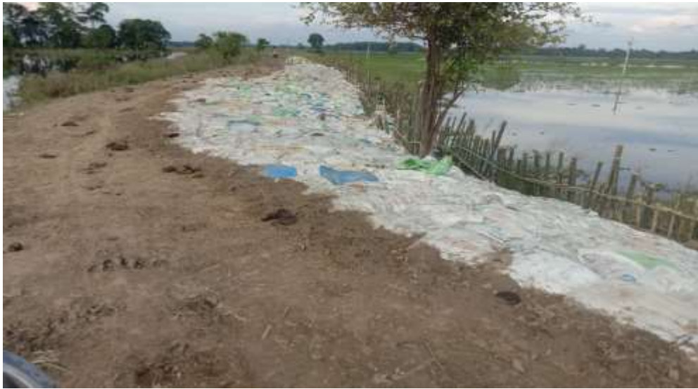
Figure 4: (a) current situation of E-10 (Dehing bund from Bhogamur to Sessamukh)
