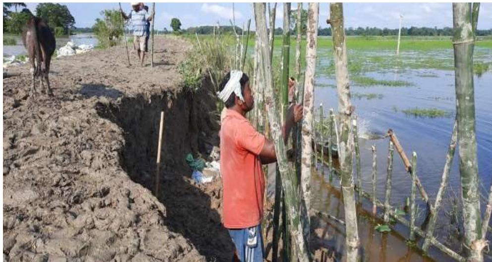
Figure 5: (b) current situation of E-10 (Dehing bund from Bhogamur to Sessamukh)
