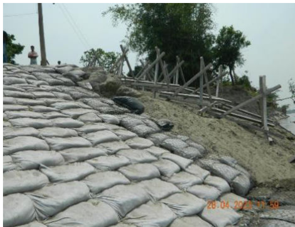
Figure 2-3. Use of Geo textile bags for Existing AE works.
