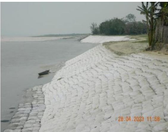
Figure 2-3. Use of Geo textile bags for Existing AE works.
