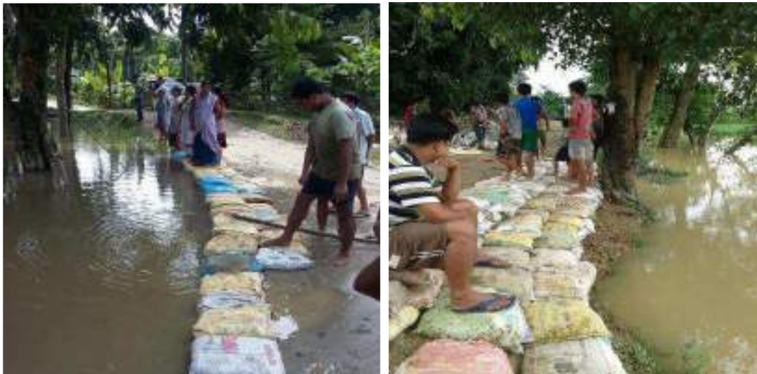
Overtopping and seepage, boiling, leakage etc.
